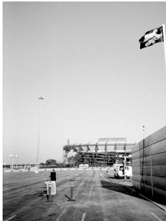
Fig. 3. Photograph of demonstration soundwall (parallax evident), Edison Field, Anaheim.
